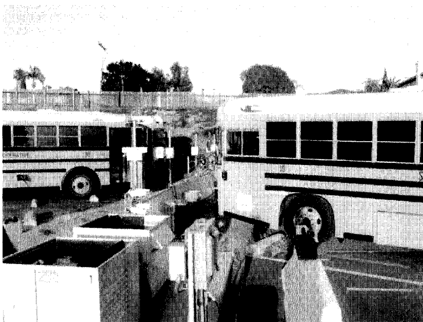
Photo of time-fill CNG refueling facility for school buses at the San Dieguito Transportation Coop - Encinitas, CA
