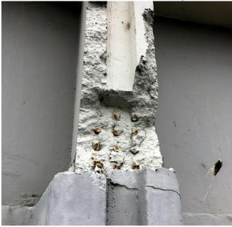
Lightweight aggregate and sand aggregate mortar visible (note ledge of integral beam that provides vertical bearing support for the tee beams):
