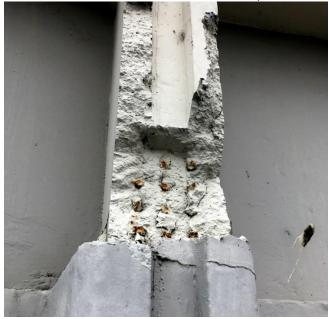
Lightweight aggregate and sand aggregate mortar visible (note ledge of integral beam that provides vertical bearing support for the tee beams):
