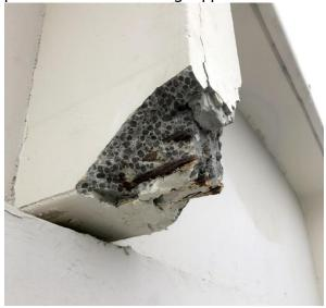
Overall picture of tee beam ends showing integral beam that provides bearing support and all damage limited to the cantilever tails:
