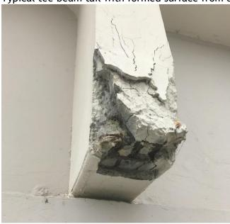
Tee beam tail with ends of tendons exposed:
